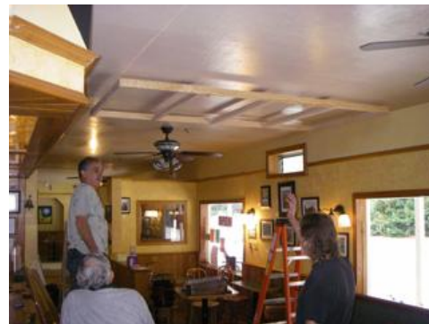
Installing the Acoustic Panels
